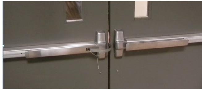
Figure 2. Typical panic bars are one of many door lock types that are vulnerable to simple, non-destructive attacks.
